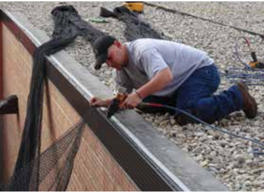
A worker installing StealthNet to keep birds out of a hospital courtyard.
