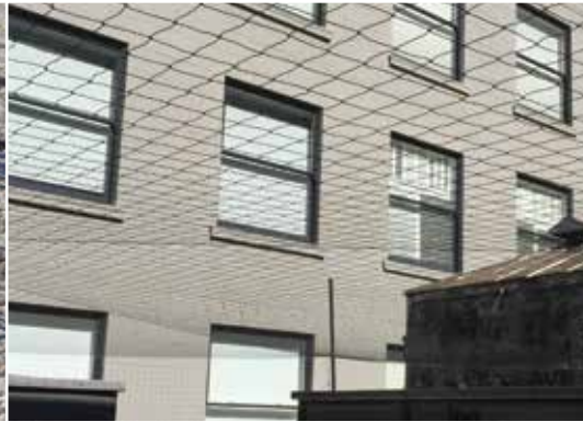
StealthNet installed over HVAC equipment keeps pigeons from entering the air space.
