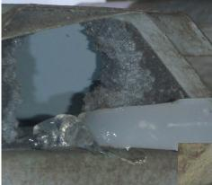
A nickel-sized dab on each sprinkler pipe joint eliminates the popular pathway. Rats had chewed the foam blockers. Rat-Out Gel is applied and blocks their travels.
