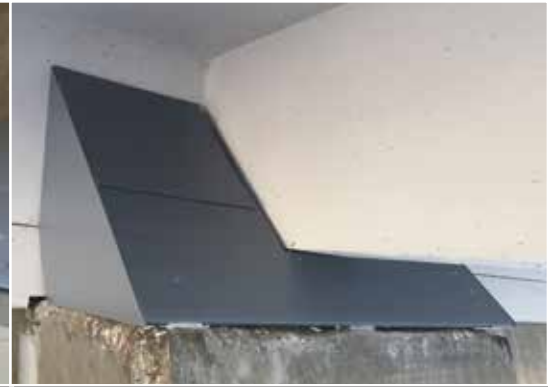
BirdSlide can be cut to accommodate beams and other architectural features.
