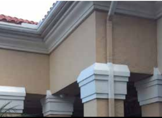
BirdSlide is mounted to these ledges and painted white to match the aesthetics of this building.
