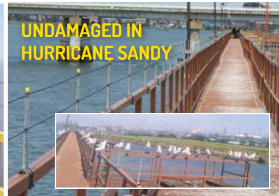
An installation on a pier to keep Gulls and Cormorants from perching
