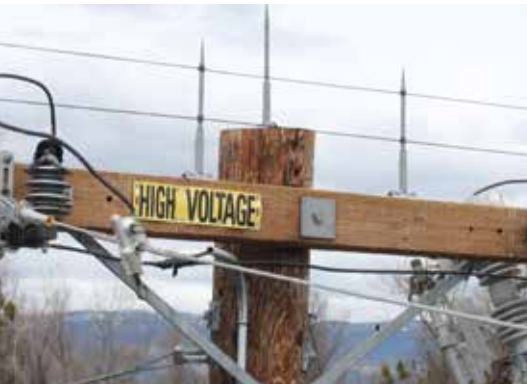
Crossarm installation to deter Ospreys.
