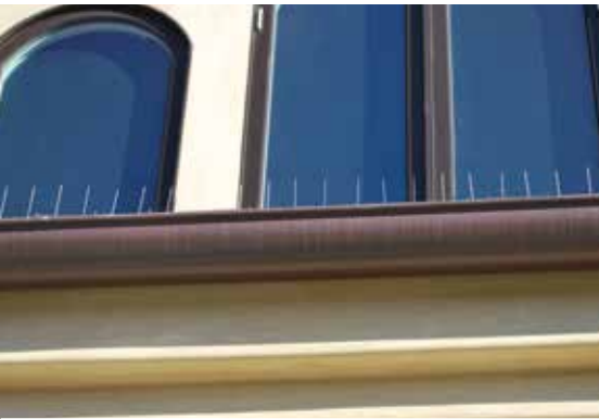
Gutter-Point is hard to see, but it's there; protecting the edge of this hotel's roof.
