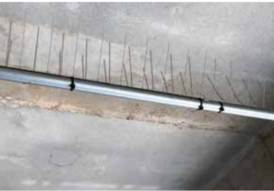
Dura-Spike attached to an electrical conduit with zip ties.
