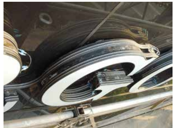
Bird-Shock Flex-Track is glued to large sign letters to deter pigeons and sparrows from nesting.
