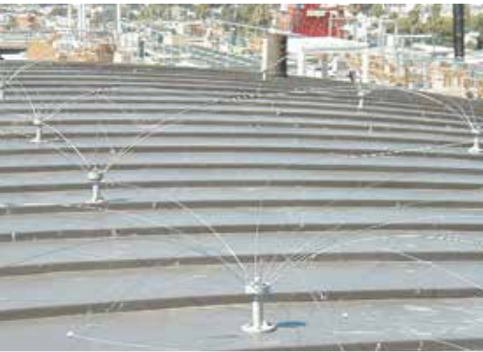
A sea of Daddi Long Legs protect a roof near the ocean from hundreds of gulls.
