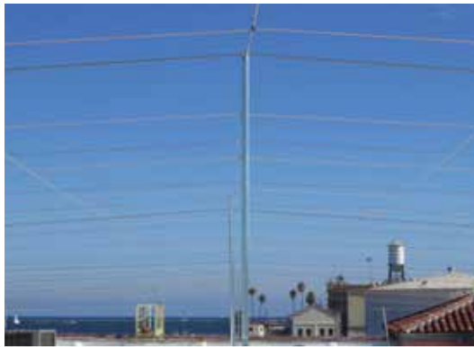
Adjustable Cable Support Poles are placed evenly across a large roof to support the wires.
