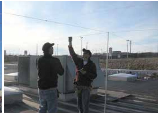
Adjustable Cable Support Poles are placed evenly across a large roof to support the wires.
