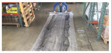
To remove the net, each operator should detach it from the structure and walk the assembly back to the staging area for disassembly.
