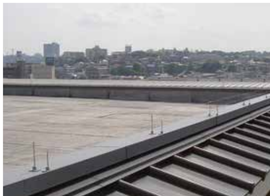
Two rows of Birdwire on this parapet cap provides low visibility protection from pigeons and large birds.
