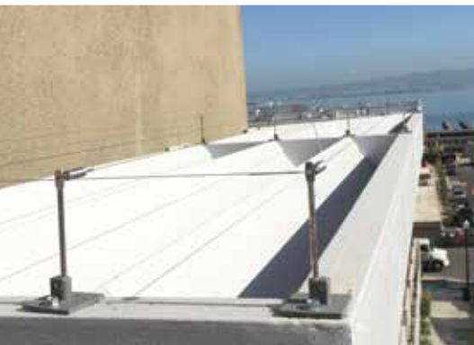
Birdwire, mounted with Glue-on-Bases screwed into this metal structure repels pigeons.
