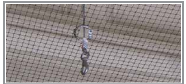
StealthNet installed horizontally under a courthouse ceiling. The cable and clip allows workers to attach banners below the netting.
