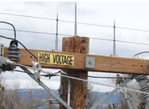
Crossarm installation to deter Ospreys.
