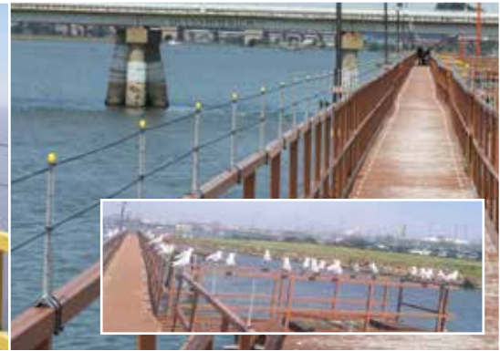
An installation on a pier to keep Gulls and Cormorants from perching
