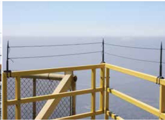
Installation on railings to deter Vultures and California Condors.
