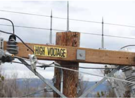
Crossarm installation to deter Ospreys.
