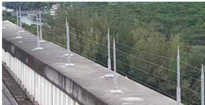
Multiple rows of Tower Guard keep large birds off wide ledges like this metal parapet cap.
