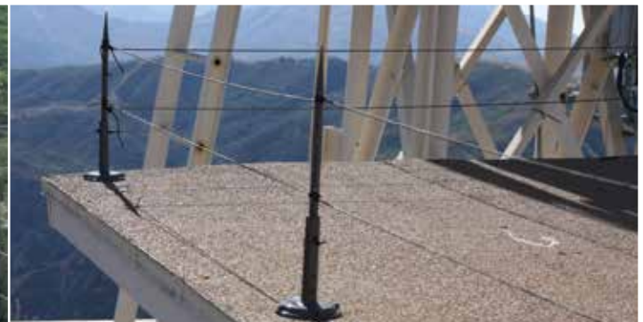
Installation on the edge of this roof repels California Condors.
