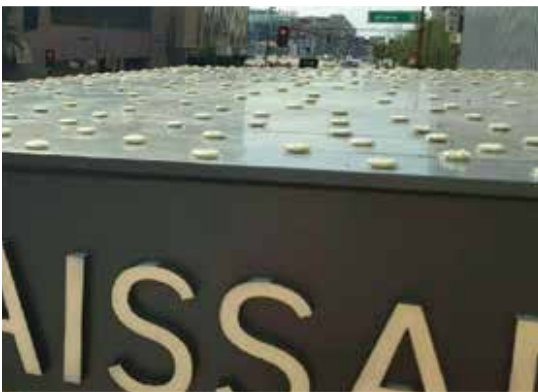
Optical Gel dishes placed strategically on this hotel's roof relocated a well entrenched flock of pigeons.
