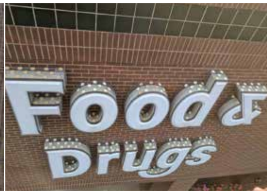
Sign letters are an ideal spot for Optical Gel because the dishes can't be seen from below.
