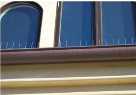
Gutter-Point is hard to see, but it's there; protecting the edge of this hotel's roof.
