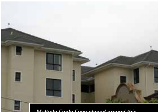
Multiple Eagle Eyes placed around this apartment complex, keep birds out of the area.
