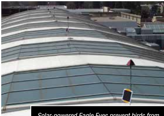
Solar-powered Eagle Eyes prevent birds from landing on the skylights of this shopping mall.
